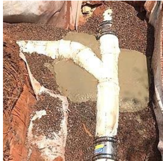
Above: Concrete thrust block at junction.
