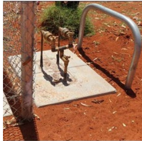
Above: Completed assembly – Duplex (W1-1-29).
