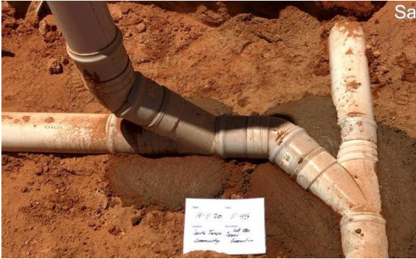
Above: Junction and thrust block installed.
