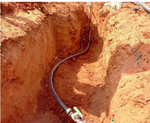
Above: Water service pipework with required loop.
