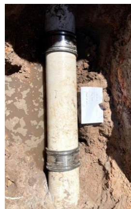
Above: Termination of old junction.
