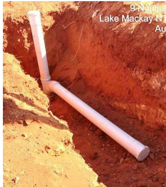
Above: Continuation of pipework.
