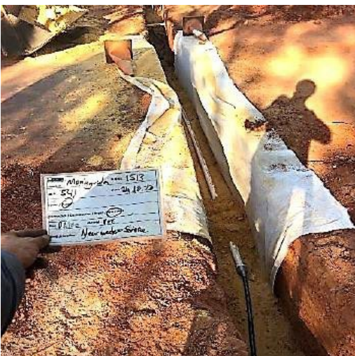
Above: Sleeve for road crossing.
