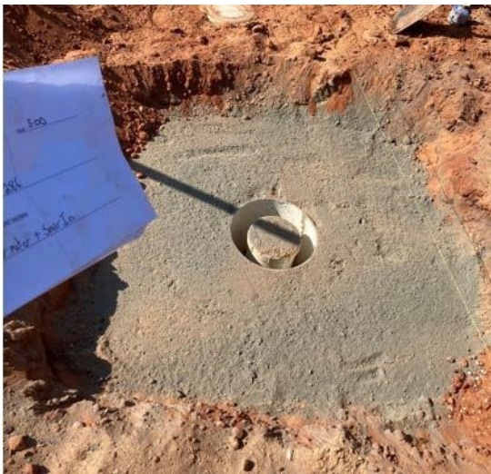
Above: Completed IO cover.
