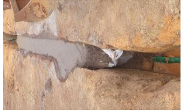
Above: Cement stabilised sand.
