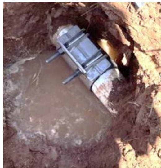
Above: Disconnection/termination showing tapping band.
