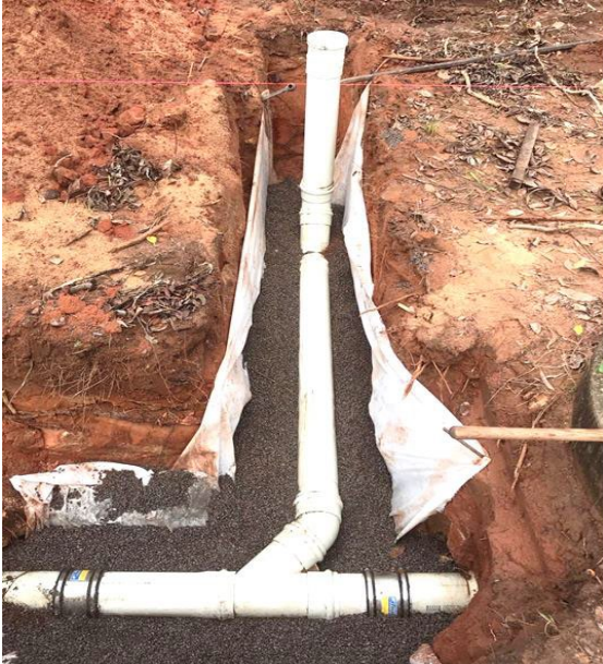
Above: Type 1 sewer connection W2-2-01 trench.
