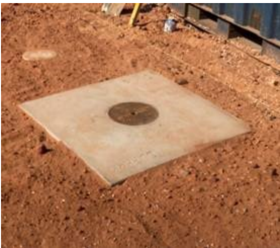
Above: Completed IO cover.
