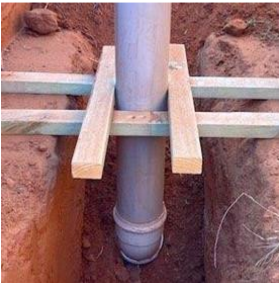
Above: Bracing at riser to maintain verticality.
