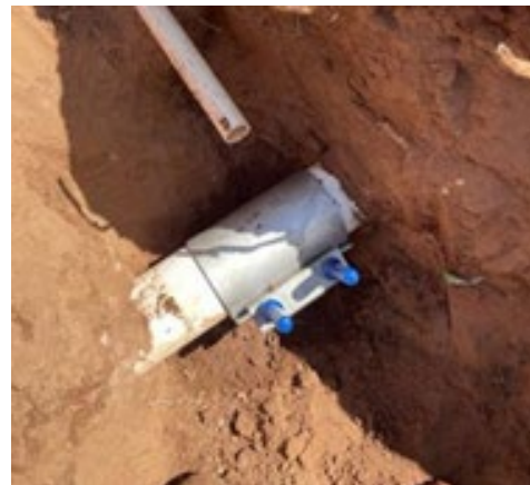
Above: Disconnection/termination showing tapping band.
