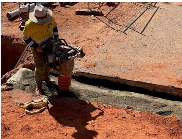
Above: Compacting of the trenching.
