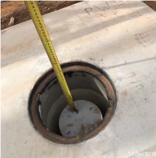
Above: Completed IO cover.
