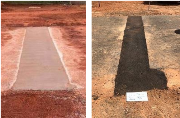
Above: Reinstatement of concrete (left) and bitumen (right).
