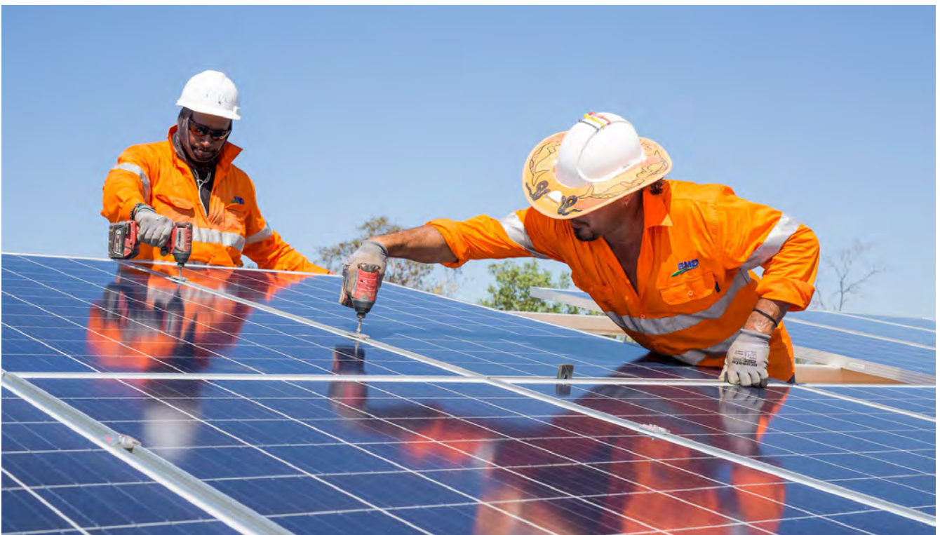
Figure 8 – Installation of solar modules at Daly River
