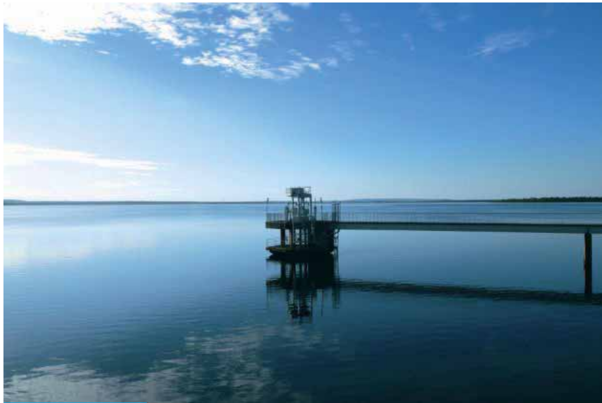
Darwin River Reservoir off-take tower.
