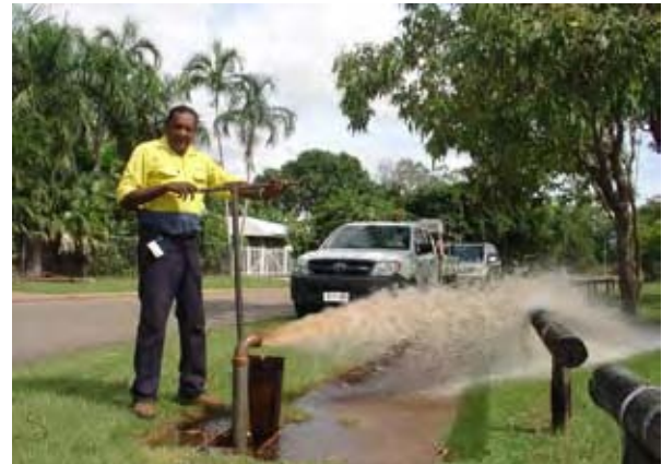
WATER SERVICE WORK FLUSHING A WATERMAIN
