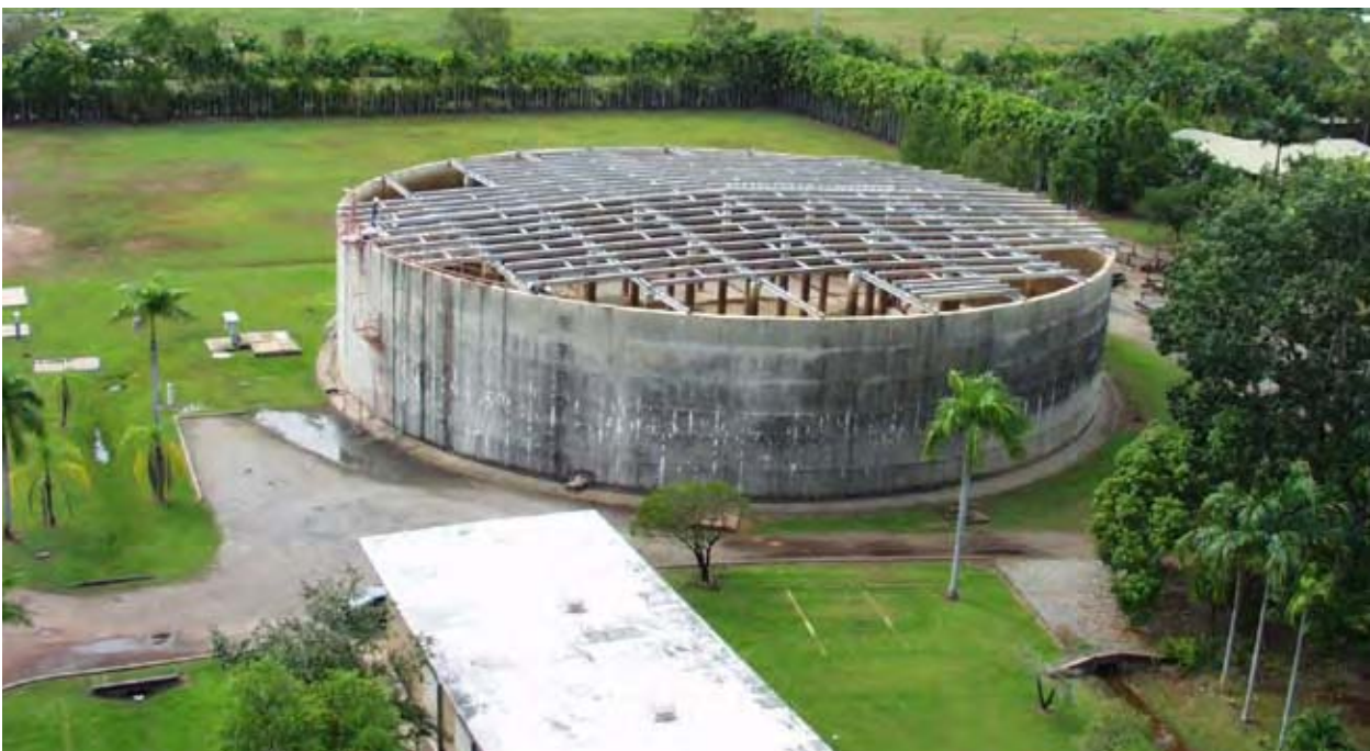
REPAIRS AND CLEANING OF KARAMA WATER STORAGE TANK
