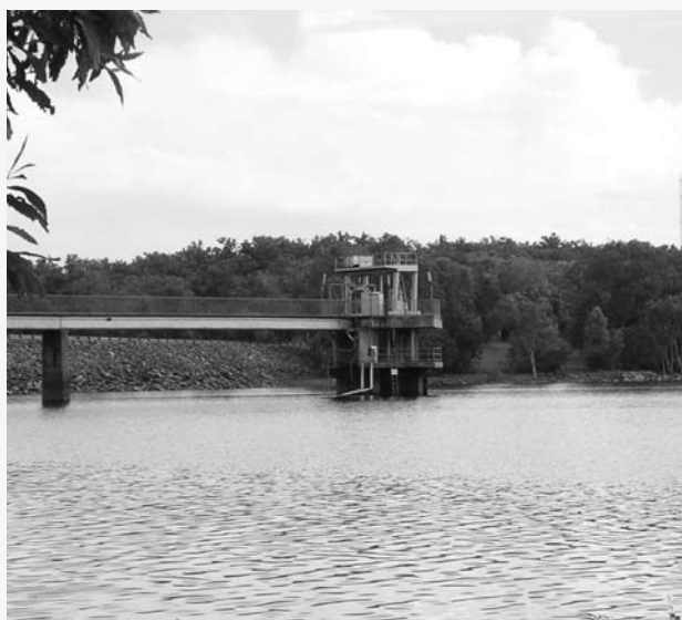
DARWIN RIVER DAM.
