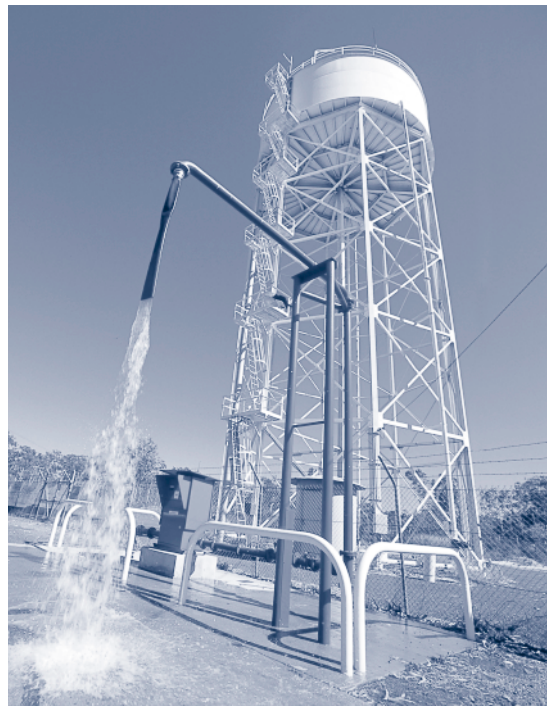
Howard Springs Elevated Tank and Watering Point.
