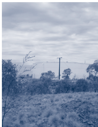
Water tank at Tennant Creek.
