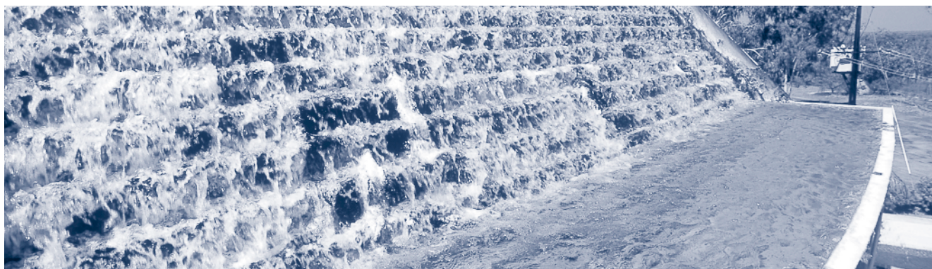
Aeration of ground water at the Katherine Water Treatment Plant helps improve water quality.
