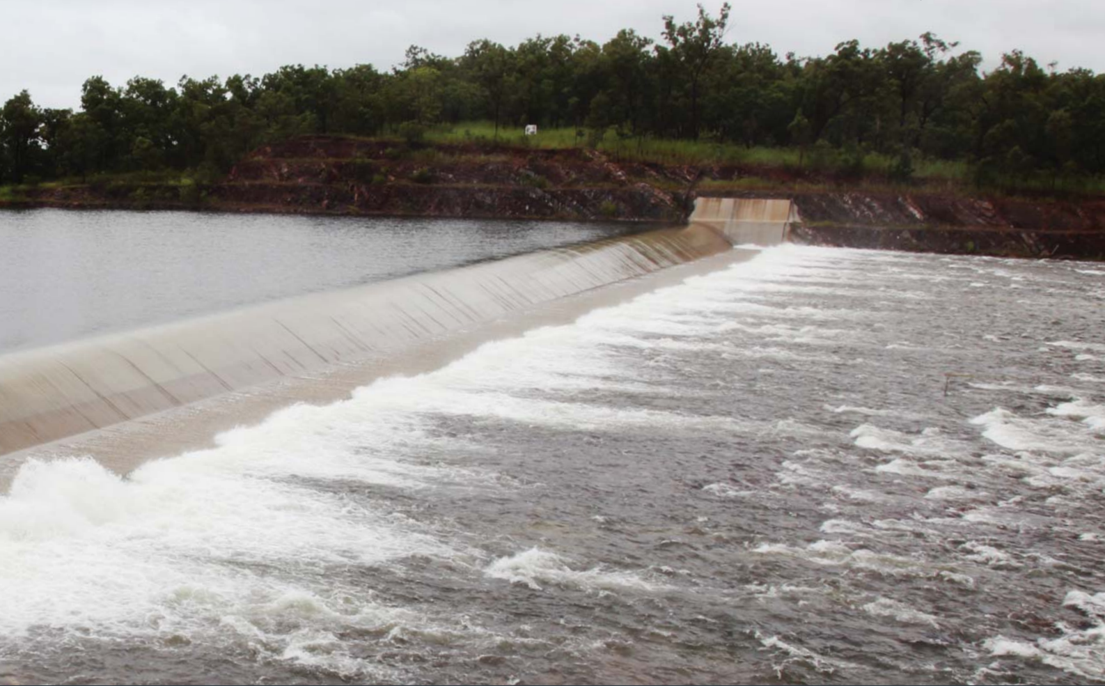
ABOVE > NEWLY RAISED SPILLWAY AT DARWIN RIVER DAM 2011
