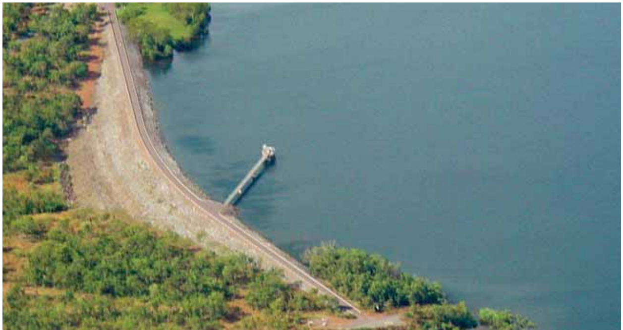
ABOVE ▶ DARWIN RIVER RESERVOIR BEFORE RAISING THE WALL AND SPILLWAY
