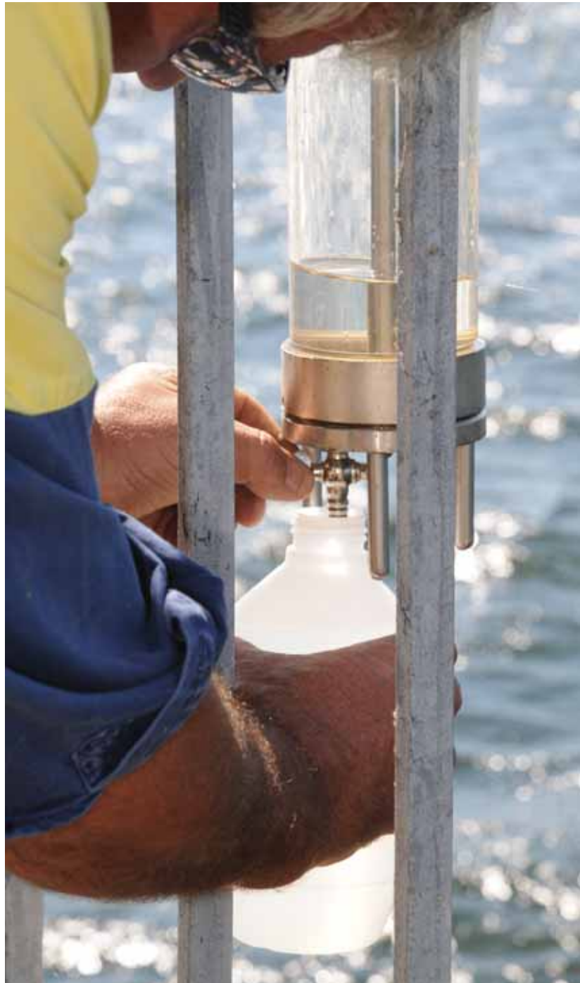
ABOVE ► WATER SAMPLE COLLECTION AT DARWIN RIVER RESERVOIR OFF-TAKE TOWER
