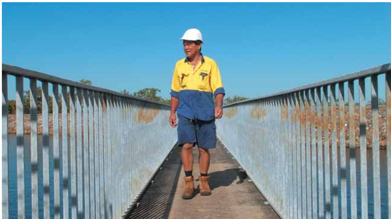
ABOVE ► WILSON LEE INSPECTING THE OFF-TAKE TOWER AT DARWIN RIVER RESERVOIR
