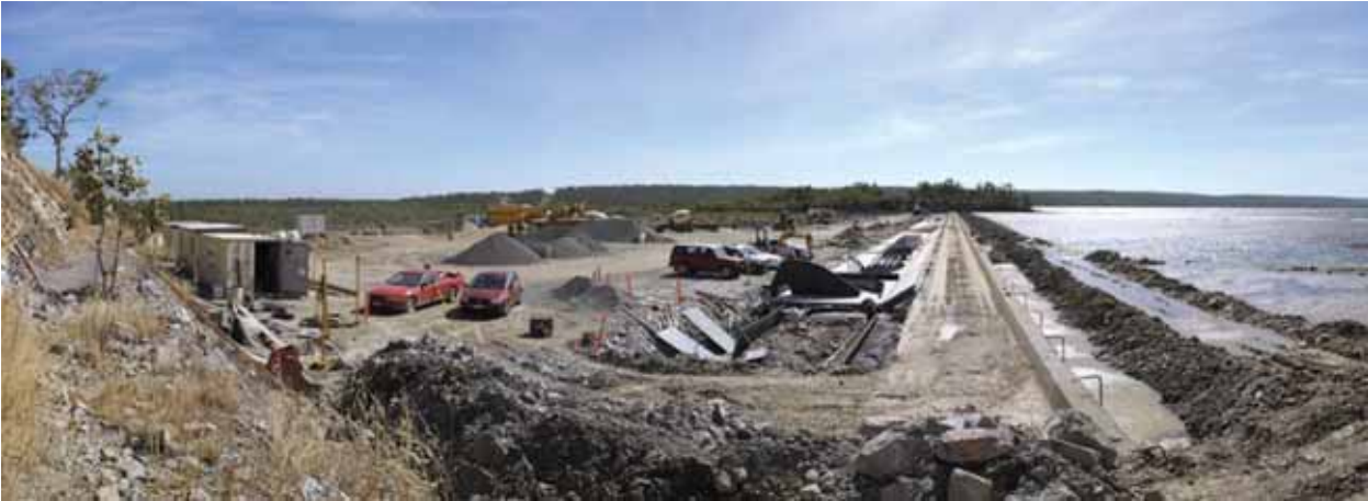
ABOVE ► CONSTRUCTION OF THE RAISED SPILLWAY AT DARWIN RIVER DAM 2010
