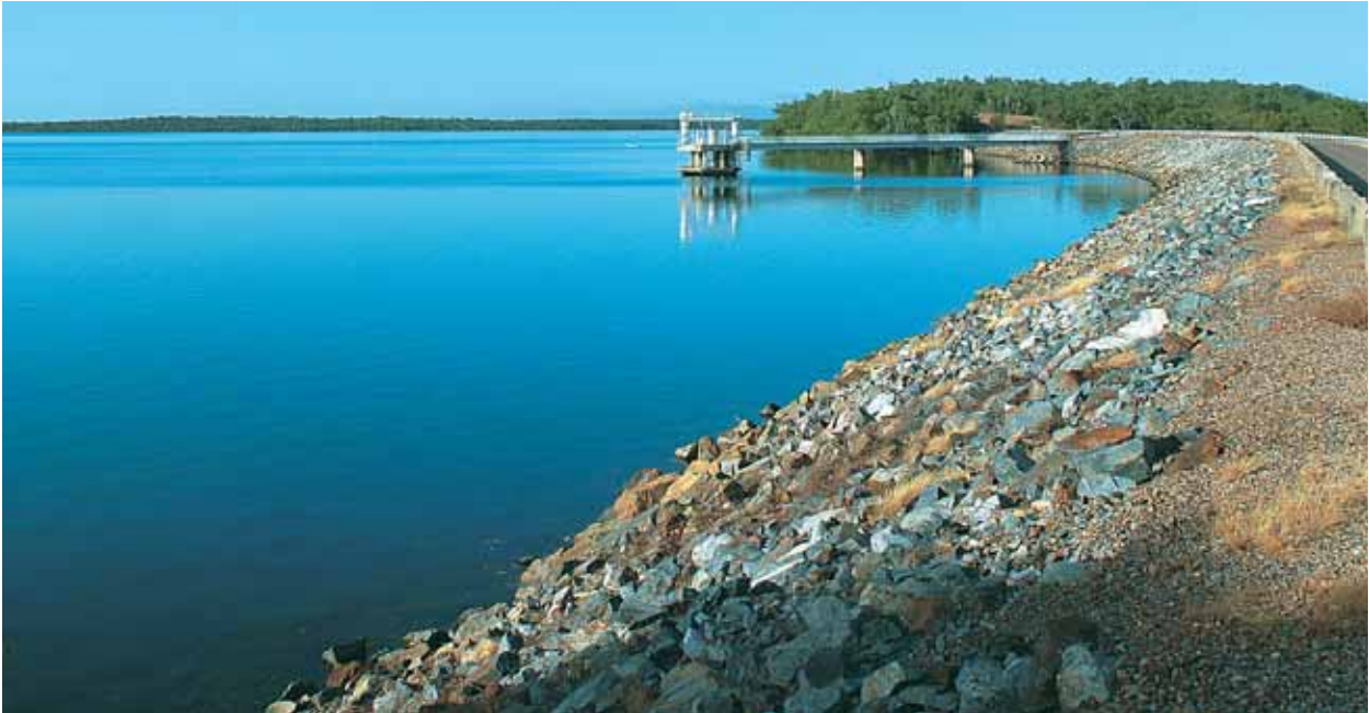
ABOVE ► DARWIN RIVER DAM WALL
