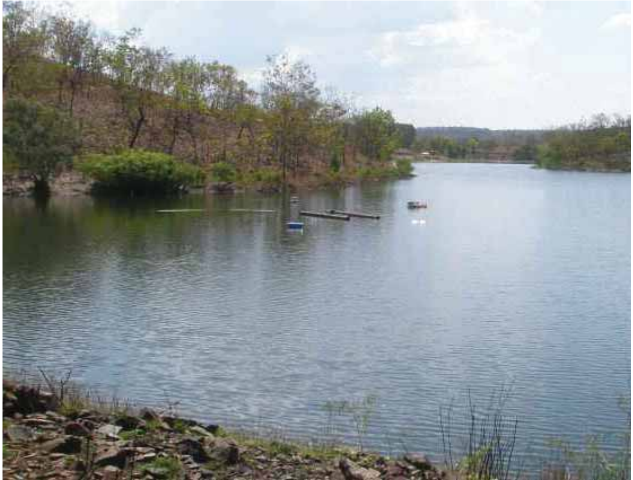
ABOVE ▶ COPPERFIELD DAM RESERVOIR AT PINE CREEK
