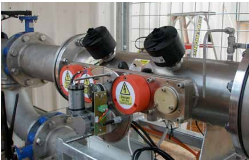
LEFT ▶ UV DISINFECTION UNIT DURING INSTALLATION IN ELLIOTT 2008
