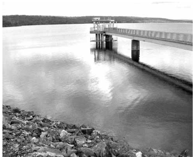
DARWIN RIVER DAM
