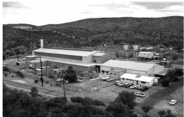
RON GOODIN POWER STATION
